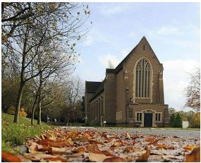
brickwork with moulded stone base and stone quoining to corners.
